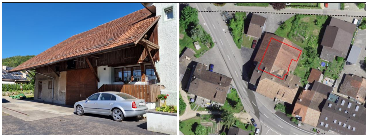
Abb. 27: Hauptstrasse 16, Scheune (Jermann AG 2023 | GeoView BL 2023)
